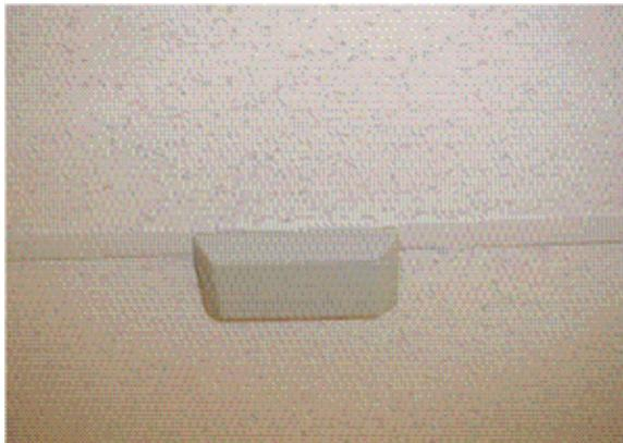
Figure 23 shows a Cisco AP1200 properly mounted to a wall.
