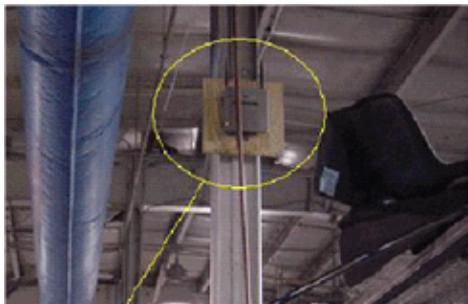
Figure 18 shows the signal propagation changes or distortions caused by an I-beam. The I-beam creates many reflections from both received packets and transmitted packets. The reflected signals result in very poor signal quality because of null points and multipath interference. However, the signal strength is high because the access point antennas are so close to the I-beam.
