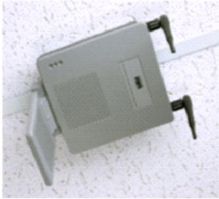
Figure 22 shows a Cisco Aironet 5959 omni-directional diversity antenna properly mounted to a ceiling T-bar. In this case, the Cisco AP1200 is mounted above the ceiling tile.
